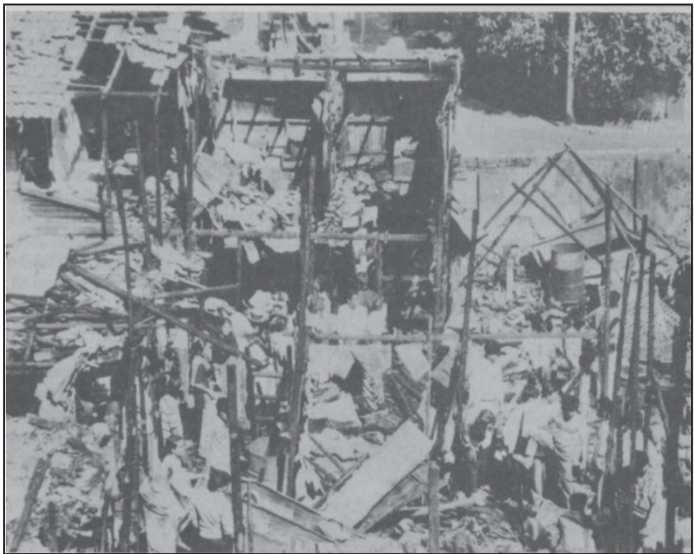
Burnt out houses in Behrampada
