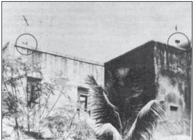
Focus lights on the terrace of building No. 30
