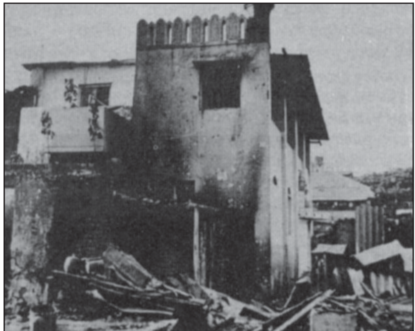
A burnt and broken mosque at Wadala
