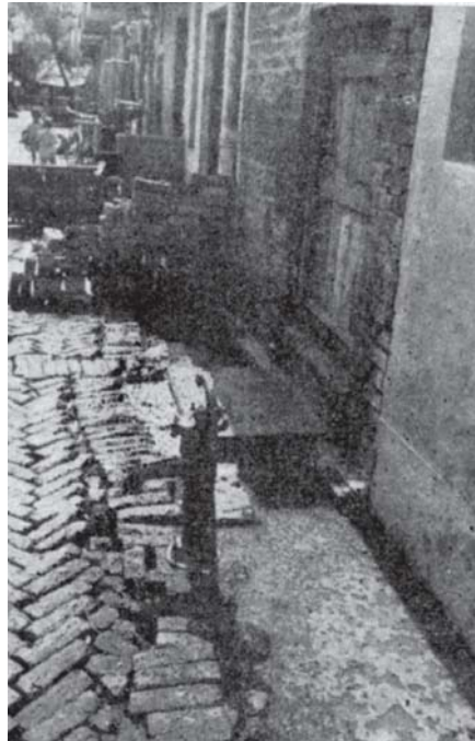
A typical water source—a handpump on the edge of a sewage filled gutter
